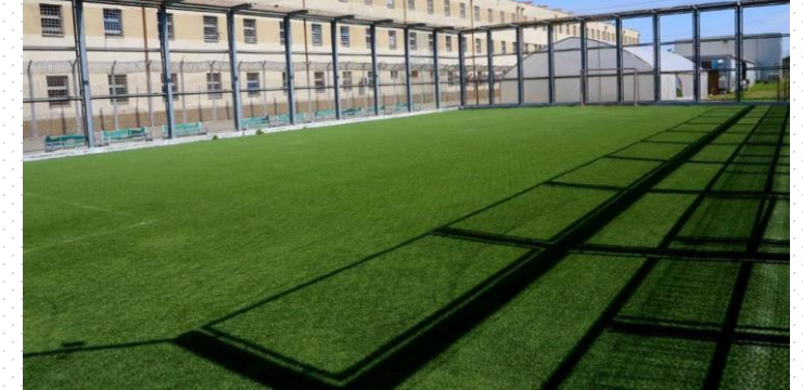
No 16 Penitentiary Facility in Rustavi
